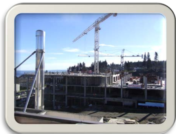
Campbell River Hospital – New Build in Progress
